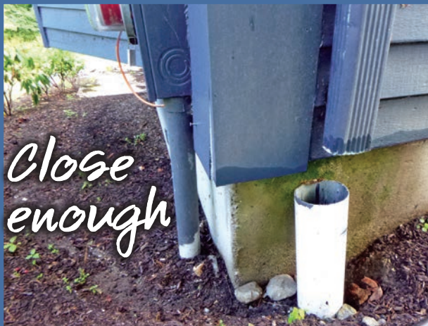
Doron Bracha | Accent Home Inspection Brookline, MA
